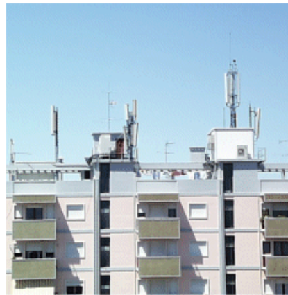
Figure 3 – BTS on the top of a building
